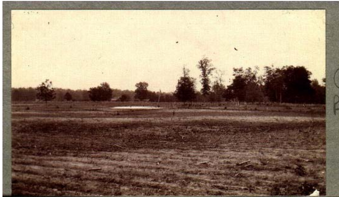
ID. FULLER, M. L. no. 137 Coalescent or linear blows obstructing drainage in the Arkansas district. Sand blows of the New Madrid earthquake, Blytheville. Mississippi County, Missouri. 1904.
